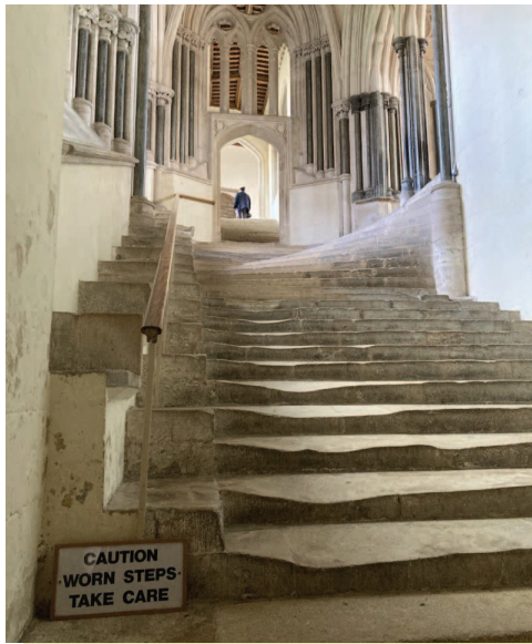
The spectacular staircase up to the Chapter House.
